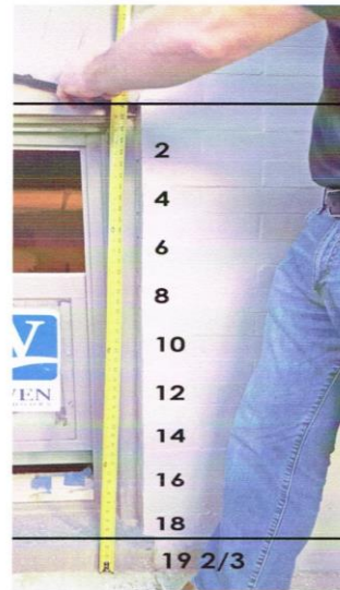
John Casey showing how he shortened the window openings by 2 1/3 courses and raised the sills 6" above their original positions March 8, 2016
